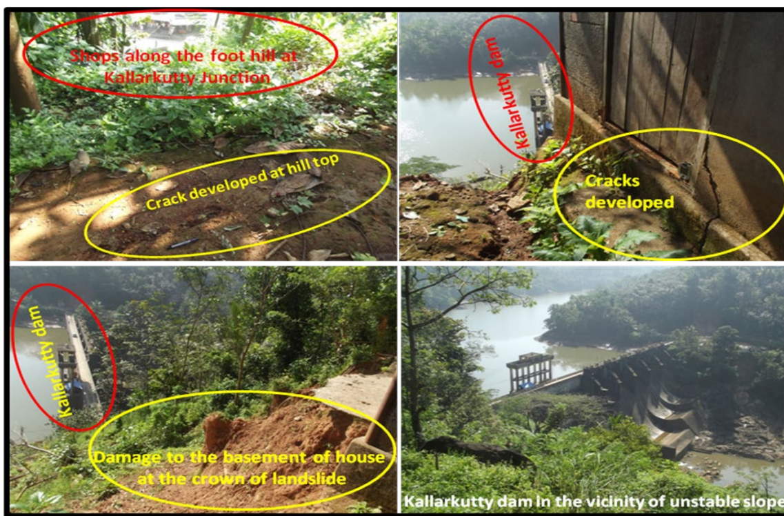
Fig. 6 Impact of landslide occurred on 5 th and 6 th of August 2013 at Kallarkutty junction
