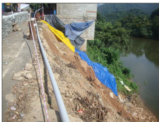
Fig. 7 Bank failure occurred between the road and reservoir on 19 th Sep., 2017
